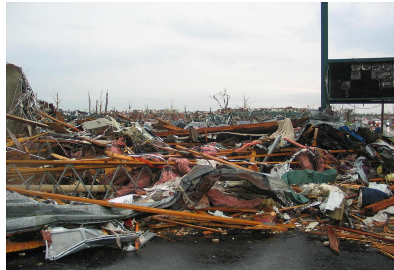
Catastrophic damage in Joplin, Missouri following an EF-5 tornado
